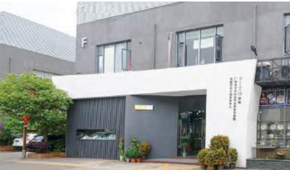
GBI / Catering Products Experience Center / Consulate kitchen
